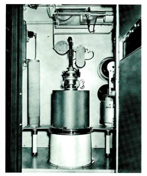
Close-up view of one of the dual final power amplifier stages. The new type 6697 tube together with grid circuits and part of the plate circuits are readily accessible from the front of the transmitter.
